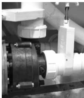
Slice Valve and Pump Union
